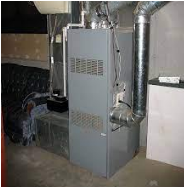
Gas furnace (contains evaporator)
